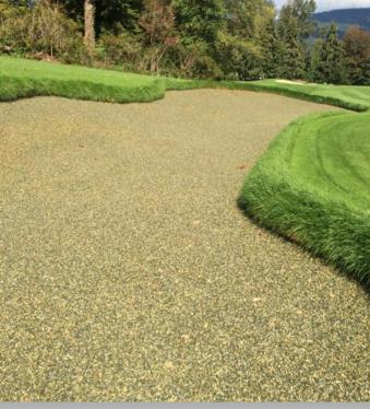
Better Billy Bunker combines pea gravel with a polymer to produce a highly porous and strong liner that works very well in wet climates.
